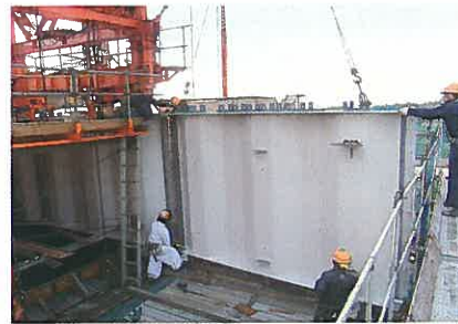
波板架設 Erection of the corrugated steel web
