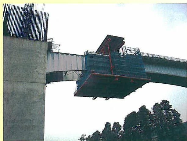
波形鋼板閉合 Erection of the corrugated steel web
