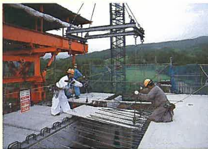
PC板架設 Erection of the PC panel
