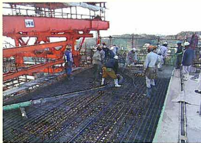
コン打設 Cast in place the concrete
