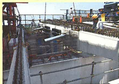
リブ架設 Erection of the rib
