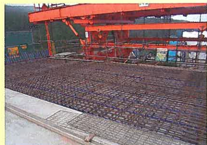
上床版鉄筋 Assemble of the re-bar of upper slab
